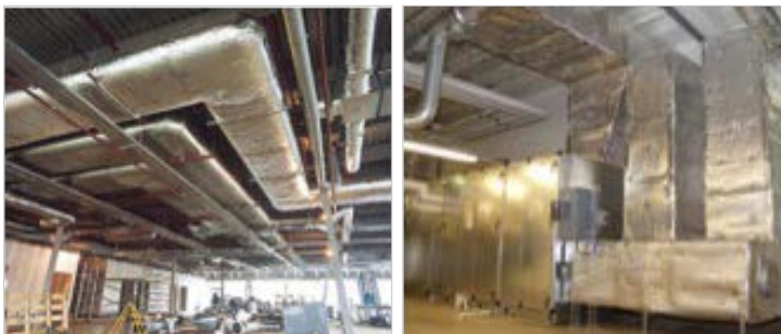
INSULATION ON HVAC DUCT WORK
